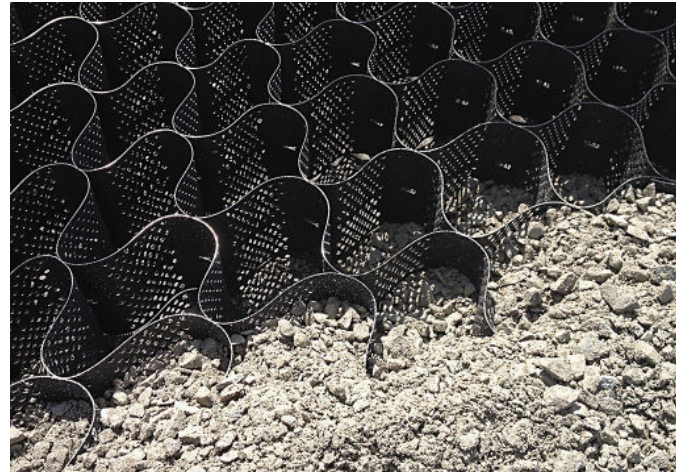
Figure 9. Geocells partly filled with aggregate
